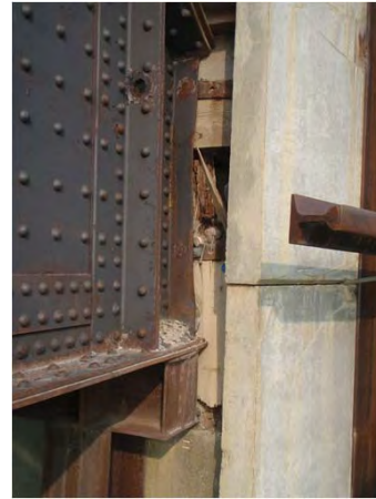
Figure 1-14: Camp end upstream ballast wall.
