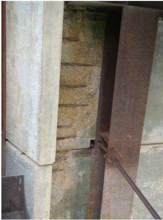
Figure 1-13: Camp end ballast wall downstream.
