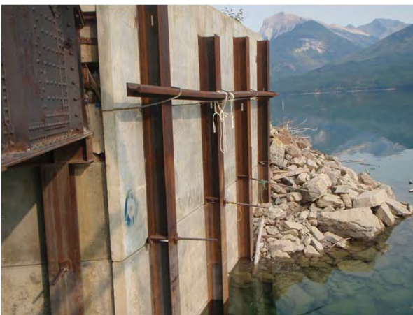
Figure 1-11: Camp end upstream wing wall.
