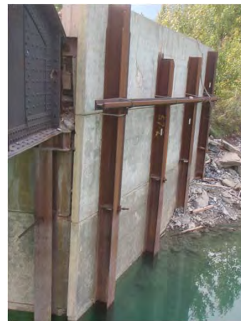
Figure 1-16: Woods end downstream wing wall.
