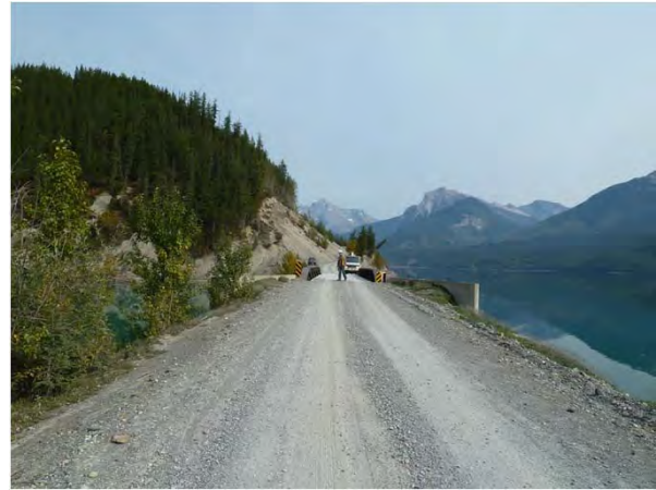
Figure 1-2: Looking towards camp end.
