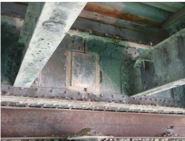
Figure 1-9: End beam splice connection.
