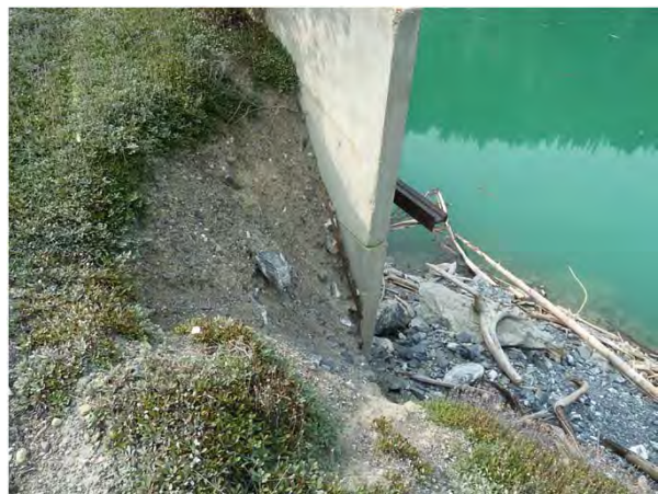
Figure 1-12: Camp end downstream embankment.
