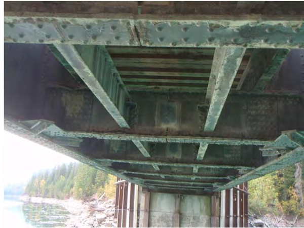
Figure 1-8: Underside of deck.
